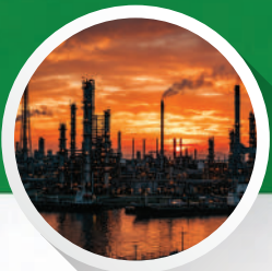
Oil & gas and petrochemical industries
