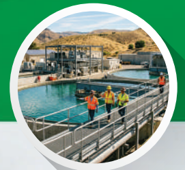
Water treatment & wastewater plants
